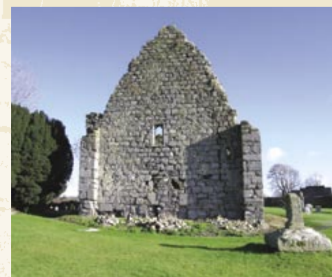
Early stone churches such as this one at Lorrha, Co Tipperary, were built in a style that copied their timber predecessors by building high steeply pitched gables with sidewalls that project beyond the gable of the church known as antae.
