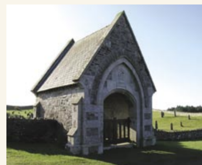
A lych gate built in 1869 marking the entrance to the military cemetery on the Curragh, Co Kildare. This is a covered gateway intended to provide shelter to the coffin and its bearers.
