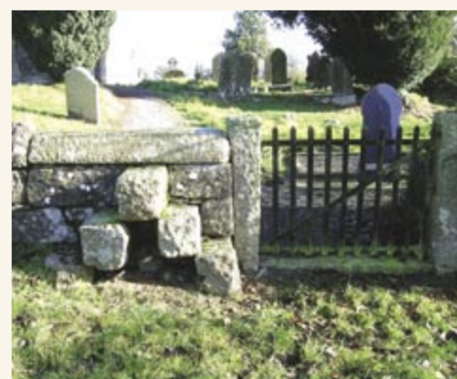
A coffin rest at Sleaty, Co Laois. Coffin Rests were built into the graveyard wall usually beside the entrance into the churchyard and are often indicated by a flat-topped wall below which, there are a series of small steps protruding from the face of the wall. It was here that the coffin was rested before entering the graveyard.
